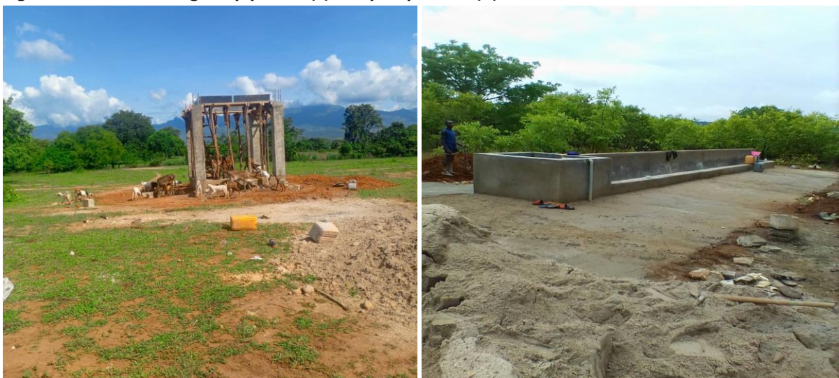
Figure 7: Photos of water tank tower (L) and completed cattle trough (R)
